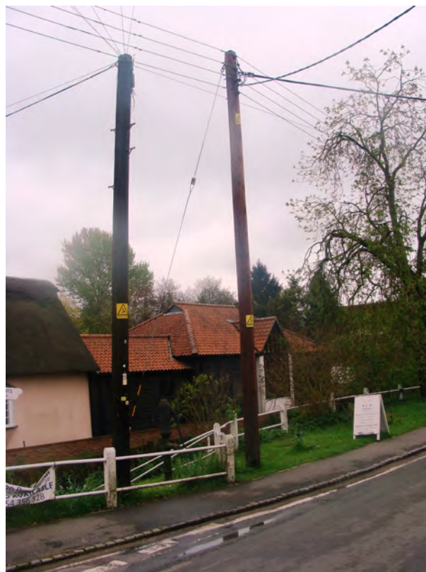
Picture 1.23 Intrusive utility poles and services in the heart of the Conservation Area.
