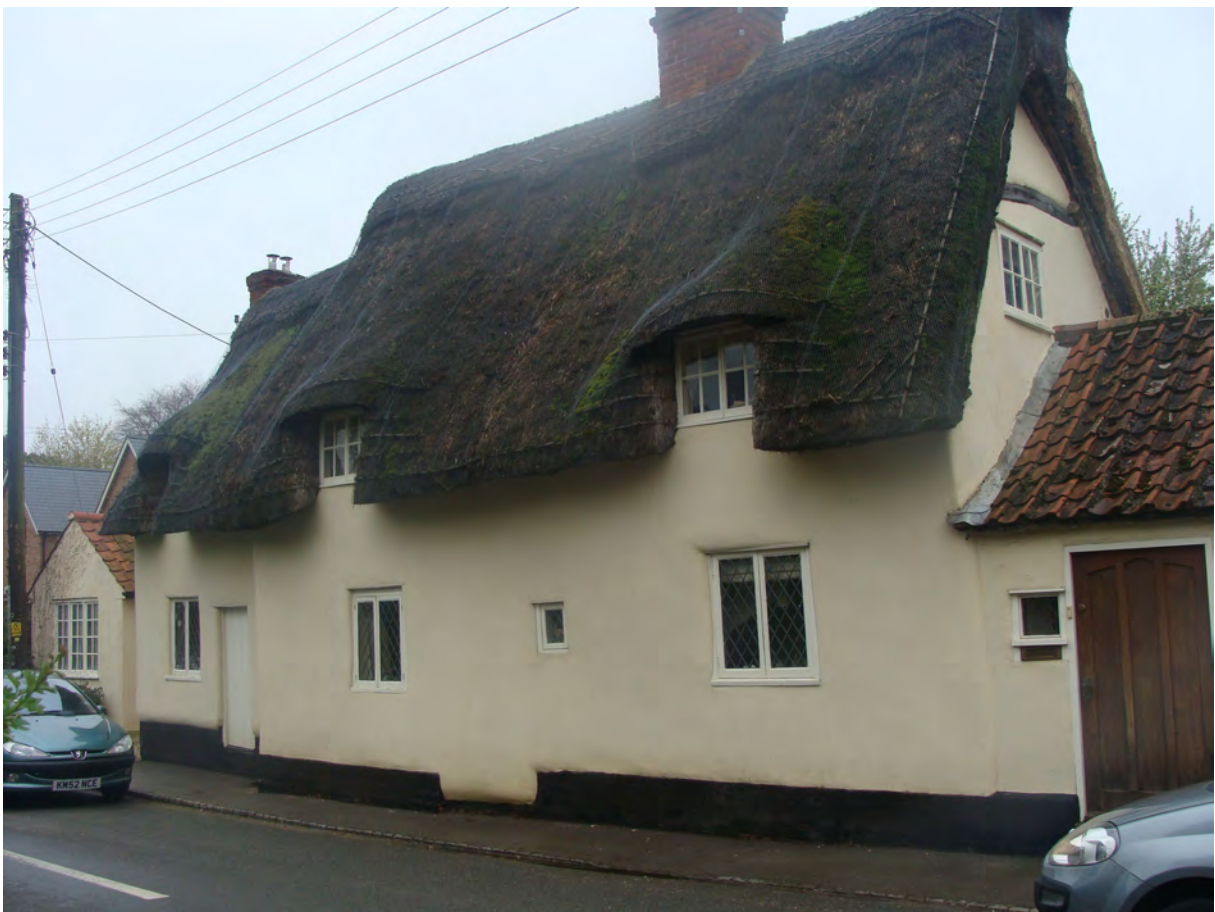
Picture 1.1 About one third of the buildings in the Conservation Area have thatched roofs
